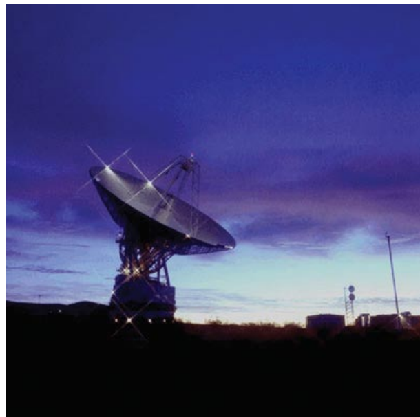
Figure 3. A radio antenna in Goldstone, CA; one of three NASA's Deep Space Network sites around the world. Spacecraft exploring the Solar System communicate with ground control using these kinds of large radio antennas. The antennas are used to both send commands to the spacecraft and receive gathered data. (Picture credit: NASA; http://deepspace.jpl.nasa.gov/dsn/gallery/images/goldstone7.jpg )
