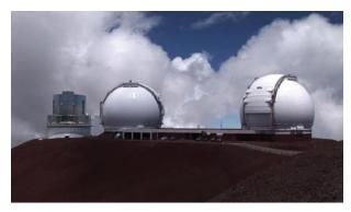
Figure 2. The Keck Observatory in Mauna Kea, Hawaii, includes two telescopes whose 10-meter mirrors are the largest in the world. The telescopes are located inside the domes seen in the figure; the domes protect the telescopes from the environment and are opened for observations. (Picture credit: NASA; http://www.nasa.gov/centers/jpl/ images/content/135066main\_Keck-9-29-05-browse.jpg)
